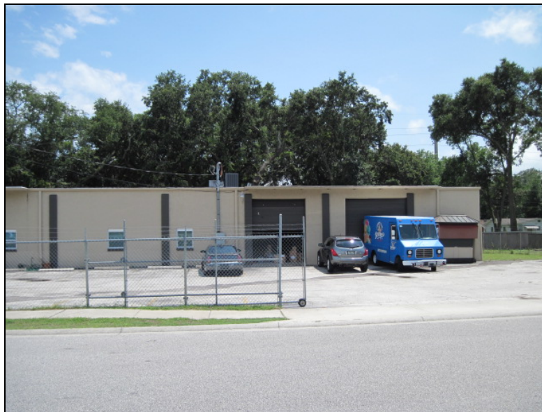
Warehouse structure to the southeast fronting both Galveston Ave. and Mill Creek Road.
